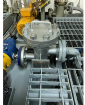
New Strainer / Filter installed
