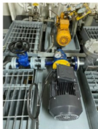
New Transfer Pump Installed
