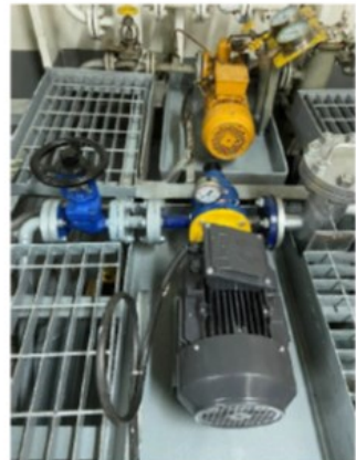
New Transfer Pump installed
