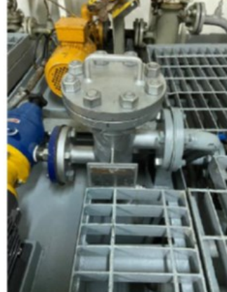
New Strainer / Filter installed
