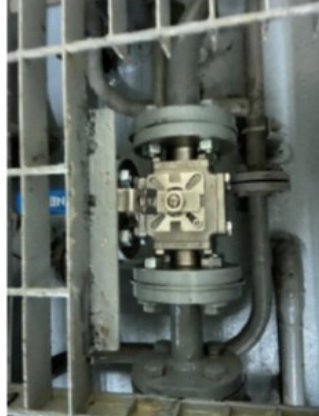
3-way valve from Storage Tank #1
